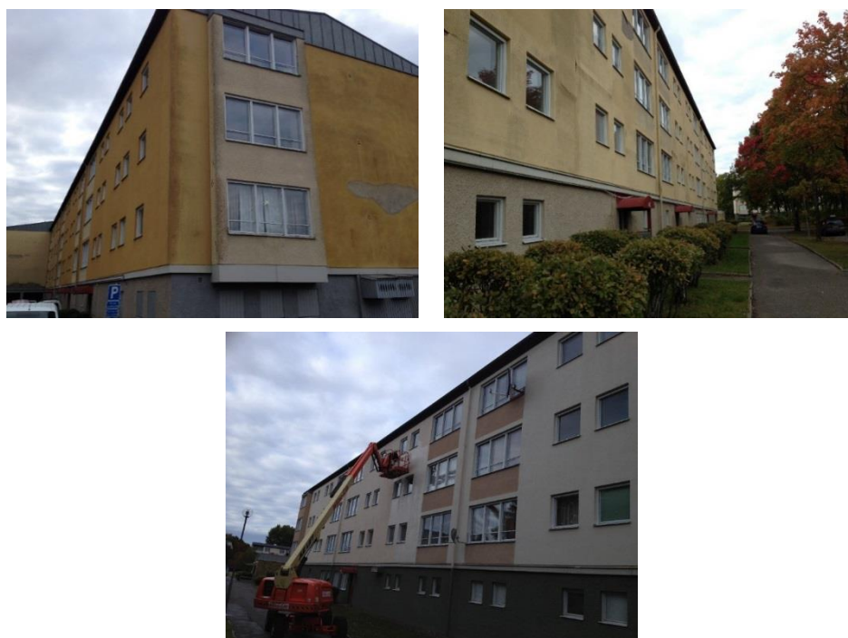
Figure 5. Houses before painting (above) and while painting after refurbishing the cracked plaster (below) Photo: Erik Dahlquist
